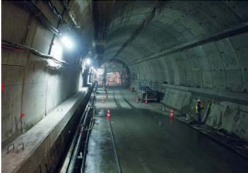
Figure 4-5 Precast Segmental lining for A-86 Tunnel, France
