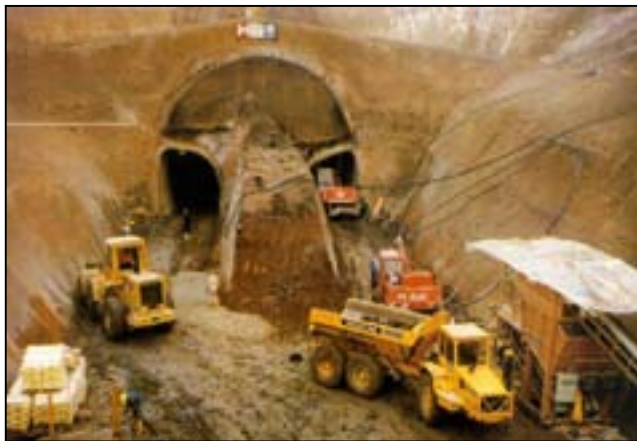
Figure 4-7 SEM Construction
