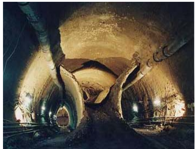
Left – SEM Portal Excavation, Right – Tunnel Drifts Excavated Using SEM
