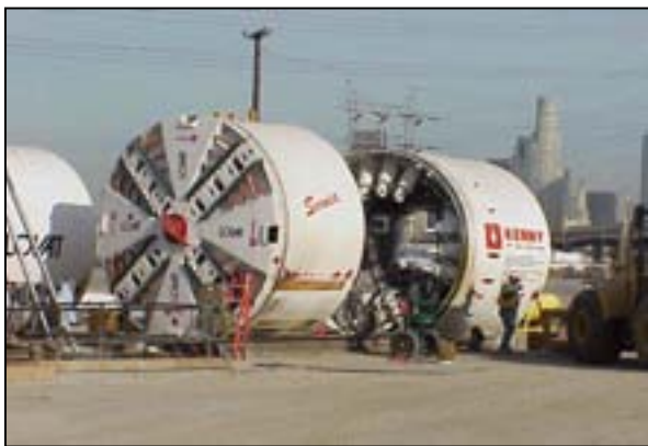
Figure 4-1 ECIS Project EPB Machine Being Assembled
