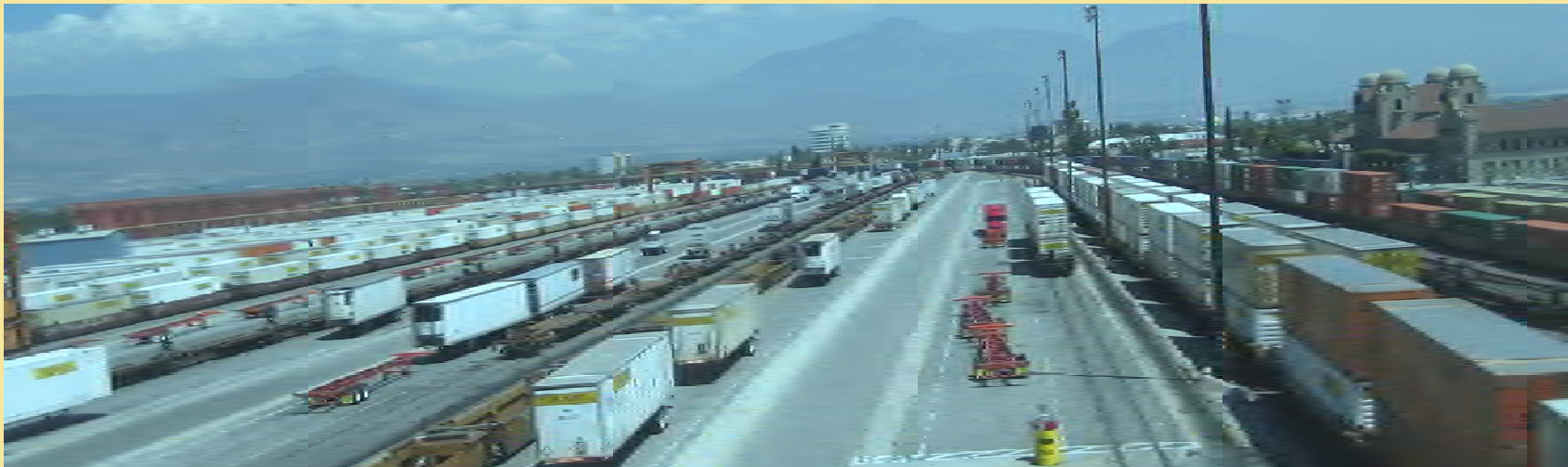
BNSF yard in San Bernardino (photo source: AECOM)
