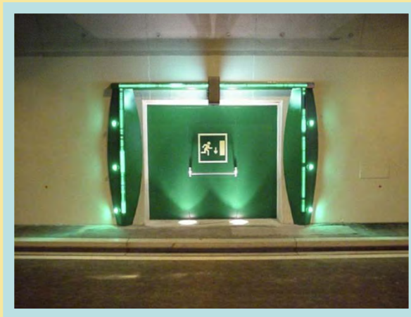
Cross Passage for Emergency Access
