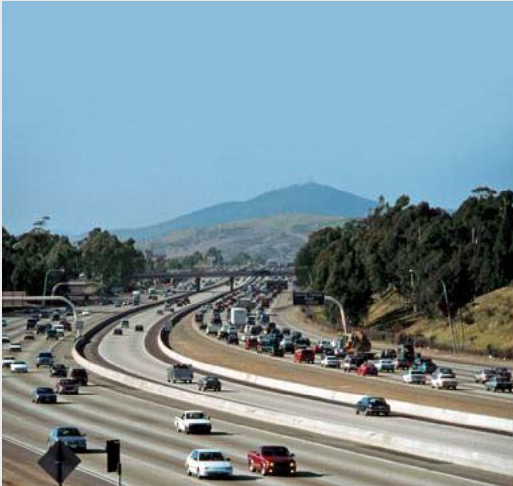
I-15 Managed Lanes San Diego County
