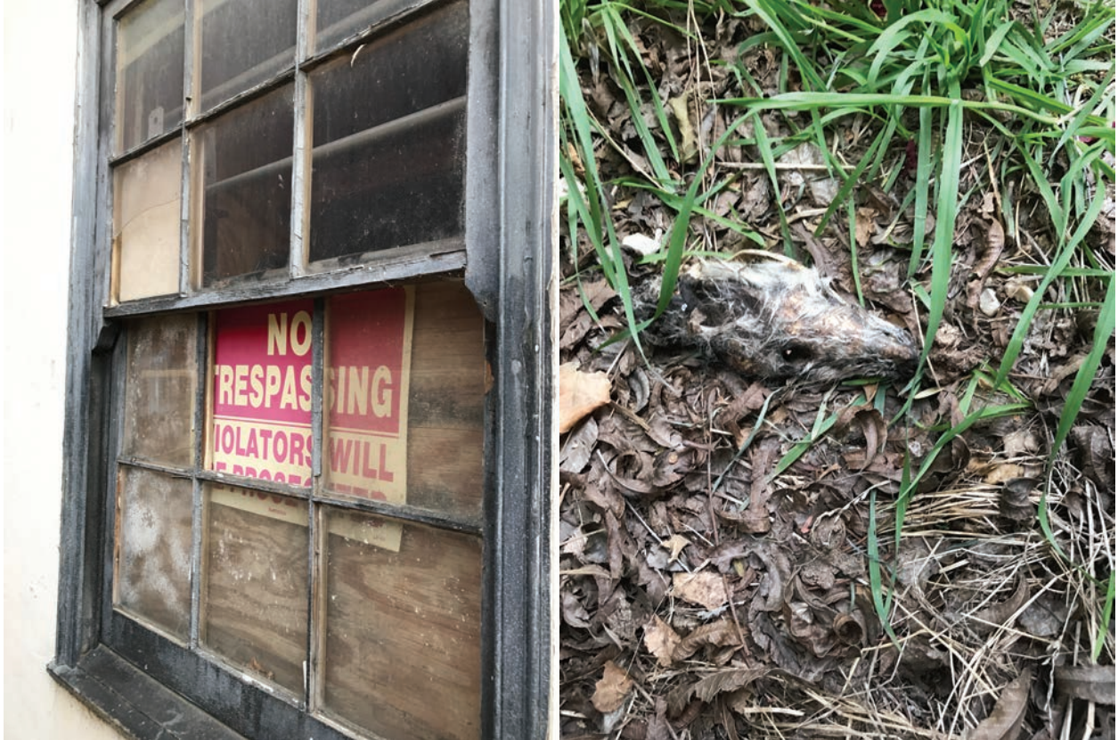
This property is where Caltrans or DCU stores excess building materials and debris. Dead rotting animals litter the property.
