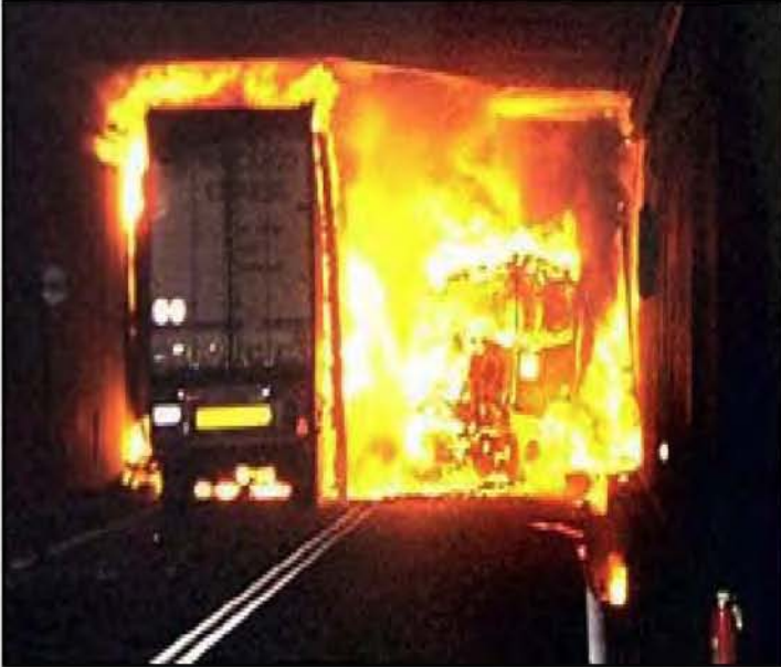
St Gotthard Tunnel Fire, Switzerland 2001 11 Dead
