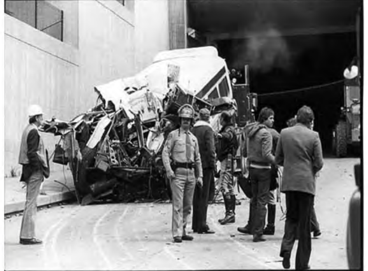
Caldecott Tunnel Fire, Oakland CA 1982 7 Dead
